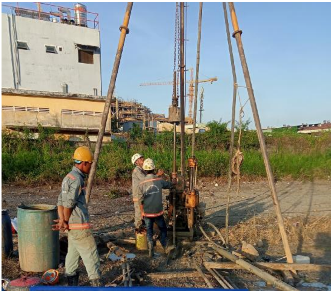
Standard Penetration Test (SPT) at bore hole HK1
